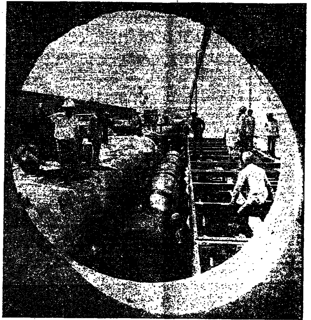
A drainage trench under construction in the floor of the main dock of the Dubai dry dock complex. The dock is being built by the Costain-Taylor Woodrow Joint Venture.
